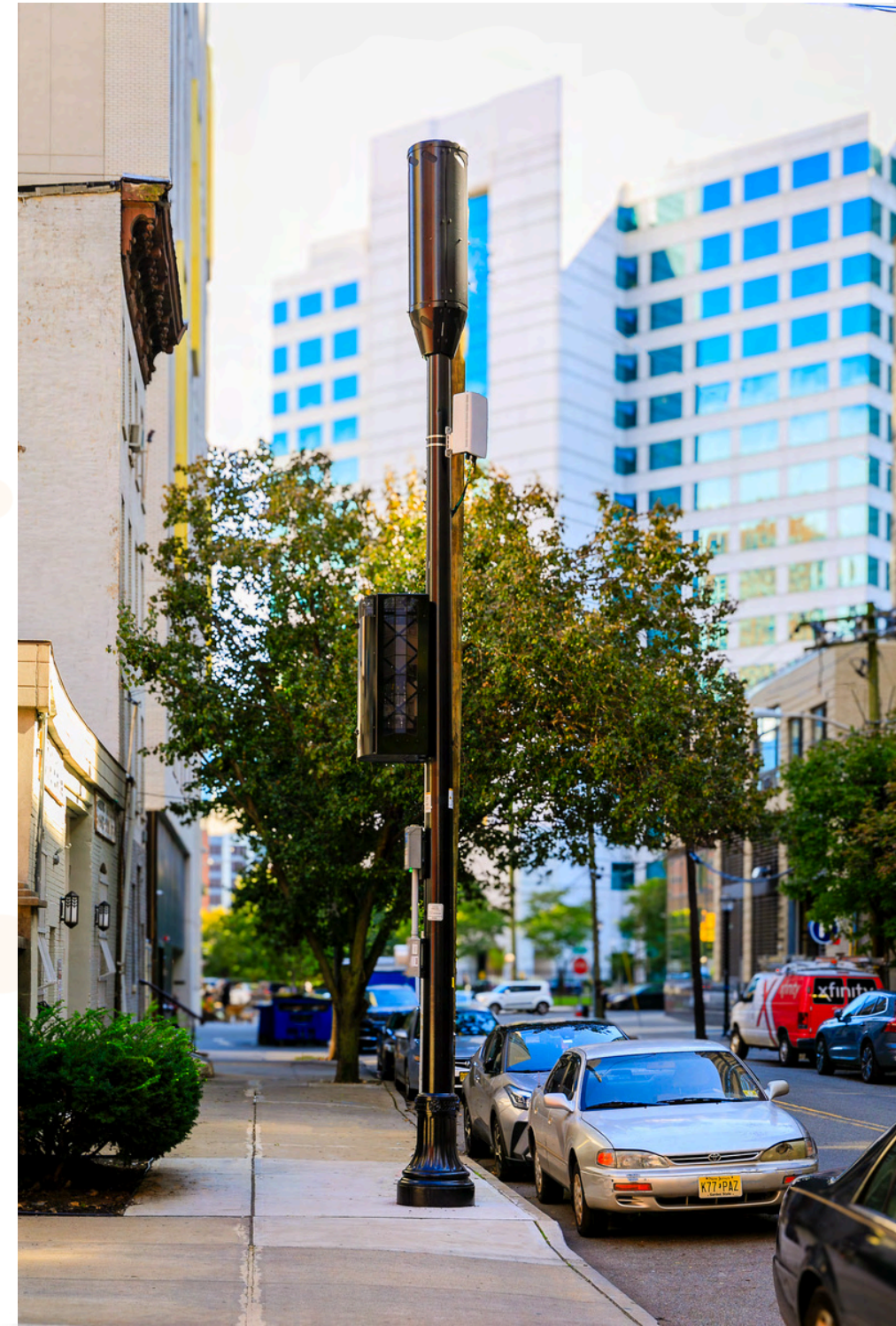
Telecom Enhanced Decorative (TED) Light Poles integrate modern telecom equipment into the municipal aesthetic landscape while meeting carrier, municipal, and local utility requirements.
